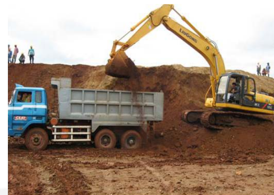
Stockpile Sorting and Loading
