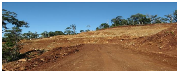
Alpha Excavation Pit
