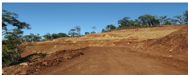
Alpha Excavation Pit
