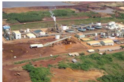
Coral Bay High Pressure Acid Leach Ferro-nickel Facility
