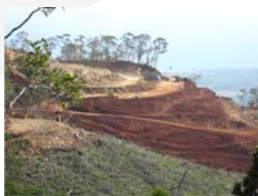
Alpha Excavation Site
