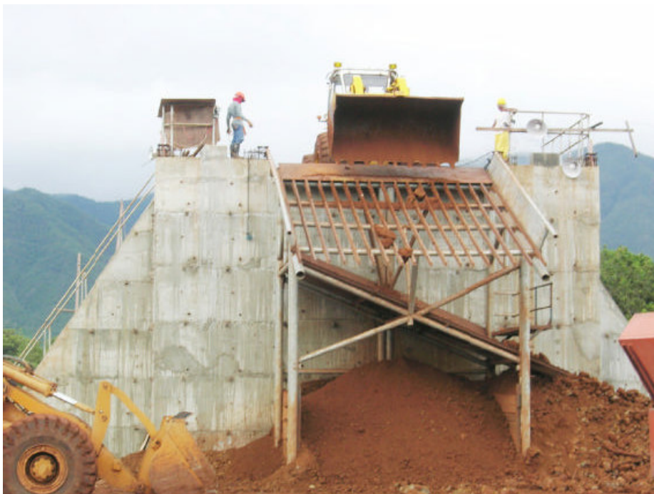
Figure 48: Grizzly in Operation at NNMDC Stockyard.
