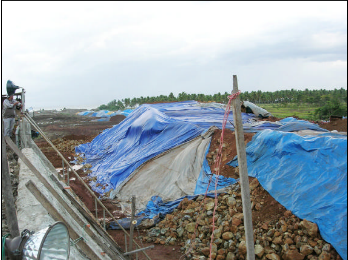
Figure 15: View of NNMDC Stockyard Looking South – Tarps Covering Material Ready for Shipment
